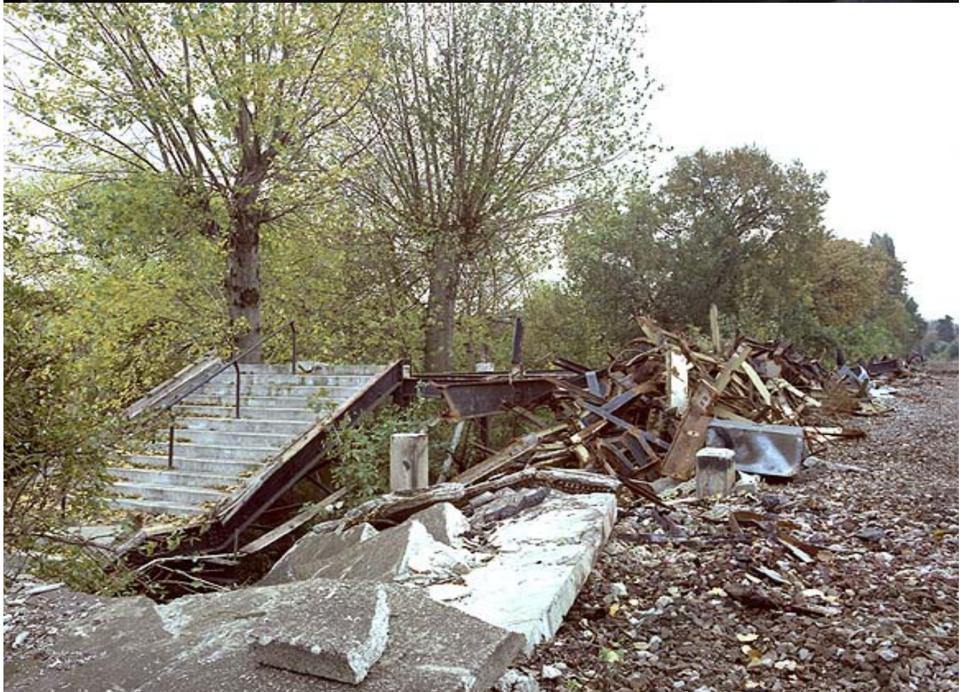
Stairs up to the platform in autumn of 1984 - shortly after the platforms were demolished
